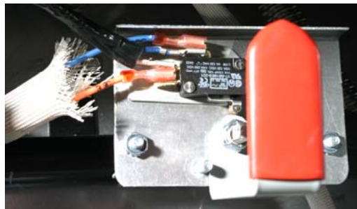
Figure 3: The wiring harness for the momentary switch is shown attached to the common (at top) and the normally open posts of the filter handle.
